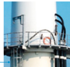
Transits for submarine cables.
