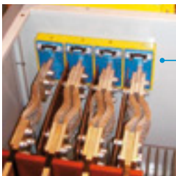
Bus bar transits for transformer room.
