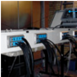
Transits for potential equalization, and standard system for control cabinets in the nacelle.
