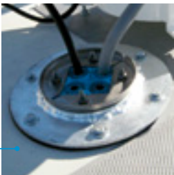
Transits for hub, radar, weather station and aeronautical obstruction lighting.
