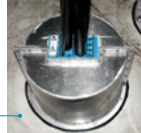
Transits for submarine cables in gravity foundation.
