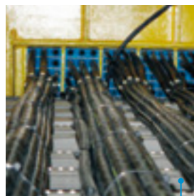
Deck transits for instrumentation.
