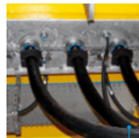
Deck transits for high voltage cables.
