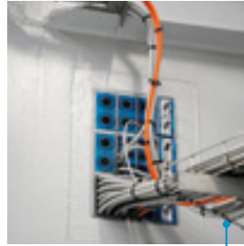
Transits between fire zones in offshore substations.
