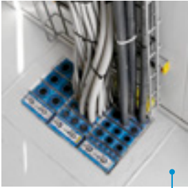
Transits between fire zones in offshore substations.
