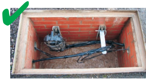
Correct standard of finished box
