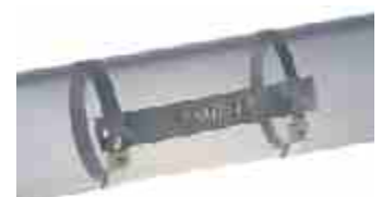
Fasten embossed tape with Ball-Lok or Tie-Lok ties
