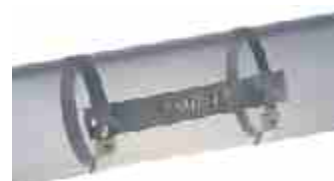
Fasten embossed tape with Ball-Lok or Tie-Lok ties
