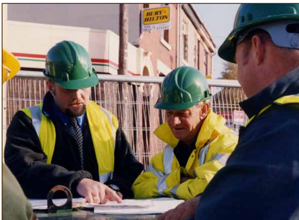
Figure 3 Discussing the work on site
