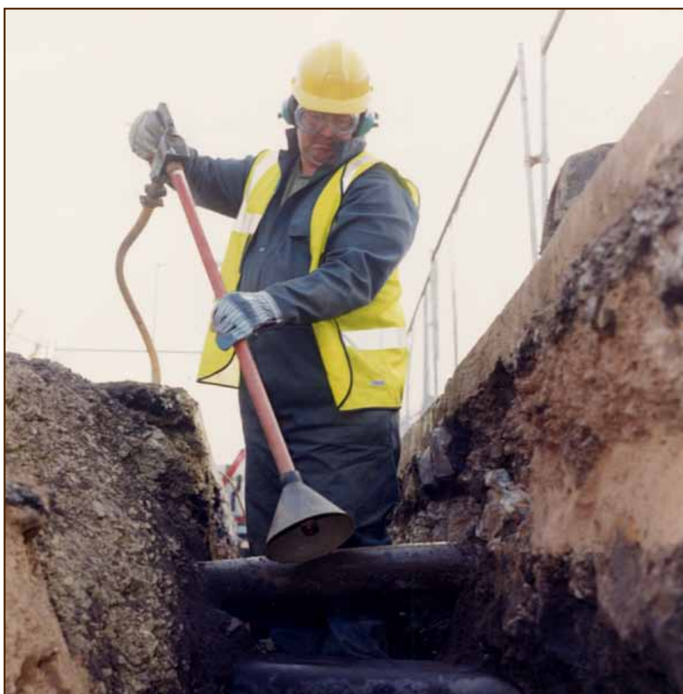
Figure 5 Using an air digging tool
