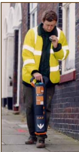
Figure 4 Using a cable locator
