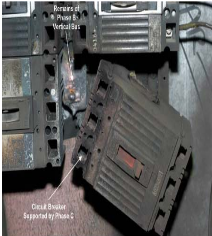
Figure 2-10. Closeup 1 of the damaged circuit breaker panel
