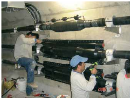
Assembling premoulded cable joints, SMPGB-C.
