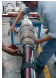
Assembly of premoulded cable joint JS.
