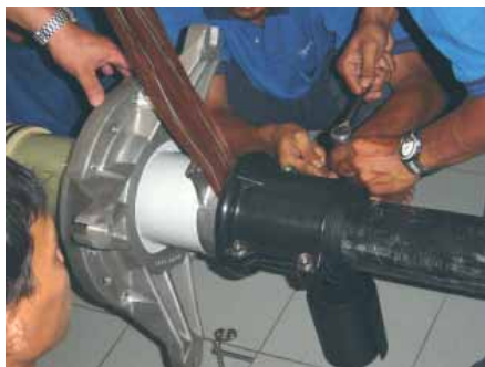
Our cable terminations can be assembled horizontally on the ground and then lifted into place, both easily and safely!
