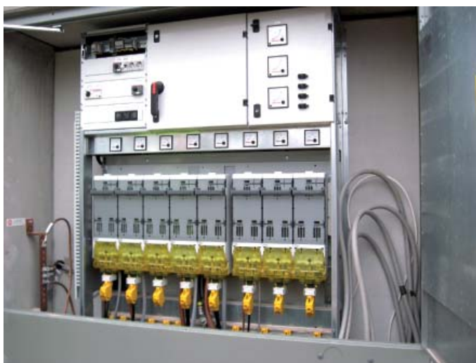
Kabeldon switching devices in a switchgear.
