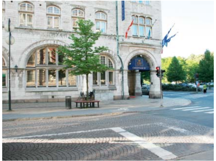
Outside the entrance to First Hotel Christian IV in Kristianstad. Cable distribution cabinet for street lighting.
