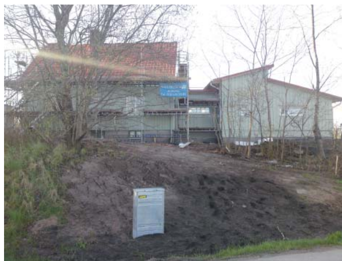
Cable distribution cabinet, Alingsås, Sweden.
