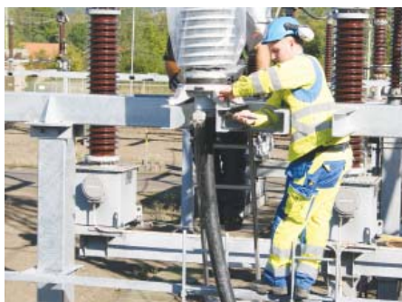
Installation of composite cable terminations, APECB.
