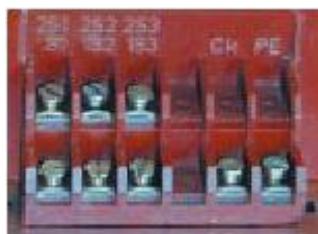
Example of current transformers terminal boxes
