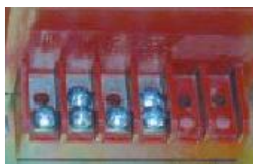
Example of current transformers terminal boxes
