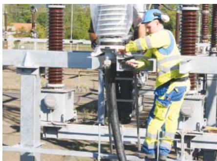
Installation of composite cable terminations, APECB.
