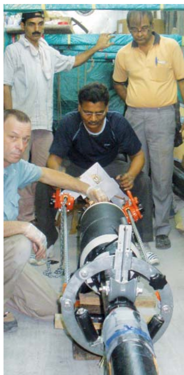
Assembly of premolded cable joint JS 245 kV.
