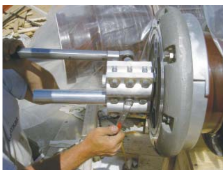
Our cable terminations can be assembled horizontally on the ground and then lifted into place, both easily and safely!
