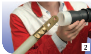
2 Place the 3M™ Cold Shrink termination body over the cable end and position at the correct point on the cable
