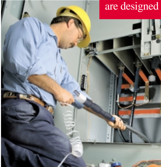
Cold Shrink QT-III Indoor Termination
