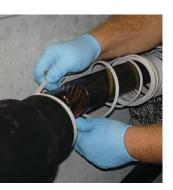
3M Cold Shrink technology has been used by the power industry for nearly 40 years, providing dependable, time-saving solutions for low to medium voltage installations. Now, this proven technology has been adapted for use in 69kV (IEEE)/72.5kV (IEC) underground cable installations.
