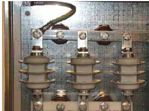
Example of link box with surge voltage limiters (SVL)
