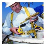
Use as a primary insulation for wire cable splices up to 600V, and for fixture and wire splices up to 1kV.
