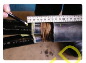
Wrap the strips of yellow stress control mastic around the crutch between the two
