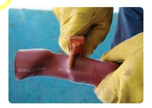
• Use a chinagraph pencil to mark the position for the sheds on the tubing at the dimension given in the termination instruction.
