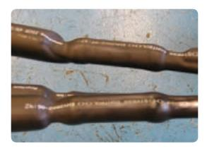
• Remove the release paper from one length of the red sealant mastic tape and wrap it around both ends of the stress control tube. Overlap the tape on to the tube by 20mm and by 10mm on to the core.
