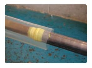
Shrink the tubing down, starting on the lead sheath and continuing towards the core
