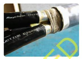
• Degrease the cores using approved solvent wipes. Make a chinagraph pencil mark on the conductive tubes 70mm from the lead sheath cut and for 20mm onto the lead sheath.
