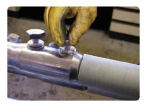
Hold the connector with the approved holding tool and tighten each bolt half a turn at a
