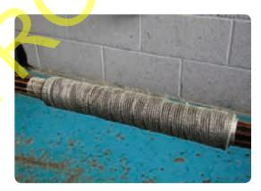
• On the cable side with the long screen wires, bend the screen wires back across the joint and form them into two separate conductors. On the cable side with the short screen wires, repeat the same exercise and fold the gathered wires back towards the joint centre.
