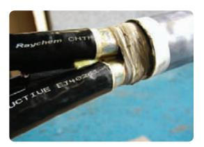
• Degrease the cores using approved solvent wipes. Make a chinagraph pencil mark on the conductive tubes 70mm from the lead sheath cut and for 20mm onto the lead sheath.
