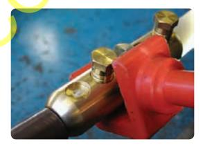
• Repeat the operation on the other side of the connector. Check that the combined tube set is located over the single-core cables and sheer off the central fixing bolt.
