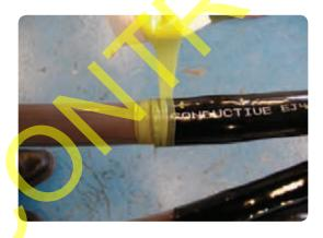
• Position a short length of the smaller diameter stress control tubing (42/16) over the core end, overlapping the conductive tubes and the yellow stress control mastic by 40mm.
