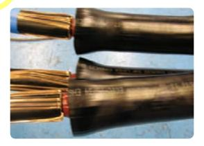
Return to each tube end in turn to complete the shrinking process completely.
