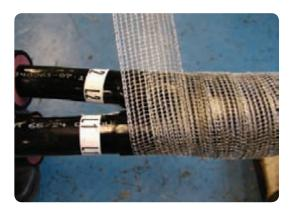
Lay the copper wire screens back across the joint and form them into three separate earth conductors. Connect the copper screen wires to each of the three earth braids using the mechanical connectors provided.
