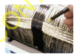
• Remove the backing from the rubber patches supplied in the kit and apply centrally (over the previously made marks) with the sticky side out.
