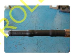
• Use one layer of red mastic around each end of the installed stress controlled tube 60mm in from each end and with a widteh of 10mm.
