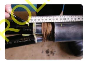
Wrap strips of yellow mastic around the crutch between the two chinagraph pencil marks.
