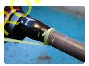
• Wrap a shorter piece of the yellow stress control mastic around the polymeric screen, starting 20mm from the screen edge and continuing for 10mm on to the insulation. Stretch the tape to half its original width during the taping process.
