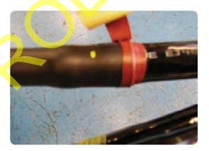
• Pull the red insulating tubes from the tube sets and centrally position them over the stress control tubes. Shrink the tubing starting in the centre before working towards each end in turn. When complete the tube should be smooth and wrinkle free.
