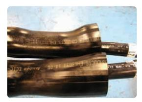
• Remove the heat from that end and start shrinking from the middle towards the other end of the tubes. Stop 50mm from the end. This ensures air inside the tube is expelled as the tube shrinks.
