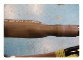
• Wrap one of the red mastic strips provided around each end of the stress control tube 30mm on to the tubing and 10mm on to the core.
