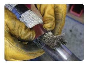
• Turn the end of the earth braids back over the two turns of the roll spring ensuring that they are flat and even. Wrap the remainder of the spring length over the braids and twist the spring up tightly.
