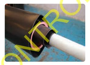
• Set the cores in their final jointing position. Check that the conductors have been cut to allow for any connector central moisture block. Remove the insulation from both conductors (3.1.3 and 3.3.7) to the connector insertion depth.
