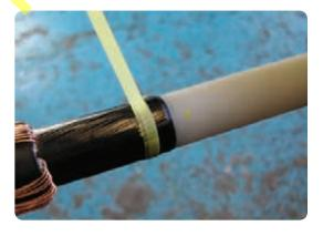
• Repeat this on the paper cable core, wrapping the yellow mastic around the edge of the conductive tubing. Cover 20mm of the conductive tubing and continue on to the clear tubing for 10mm.
