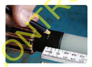
Make a second chinagraph pencil mark on the insulation 10mm from the screen cut.
