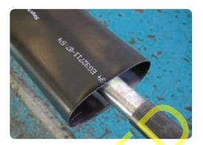
• Shrink the tubing down, starting on the tube set end and working towards the lead sheath. Once completed there should be approximately 50mm of lead sheath still exposed.
