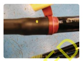
Pull the red insulating tubes from the tube sets and centrally position them over the stress
