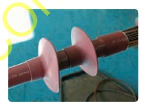
• For outdoor terminations there are four skirts to be fitted to each termination. These should be placed and shrunk into position at the measurements indicated in the relevant jointing instruction.
