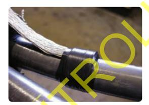
• Secure the braid ends to the armours and the support ring with a roll of tinned copper mesh sandwiching the braids between the mesh wraps.
