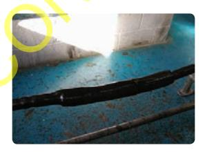
Allow the joint to cool before moving or backfilling.
