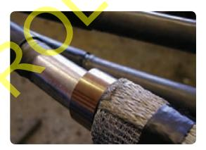
Cover the roll springs with two layers of PVC tape.
