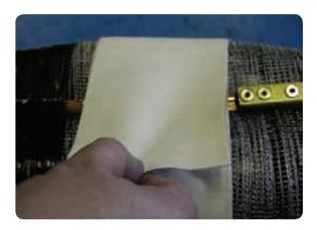
Place the two halves of the joint shell over the joint and clip the two halves together with the clips provided. Check enough clips are used to stop the resin leaking out when it is poured in.
