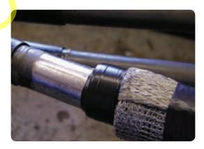
• Wrap the remaining exposed lead sheaths with the strips of red sealant tape. **This is an important moisture seal. Do not leave out.**
