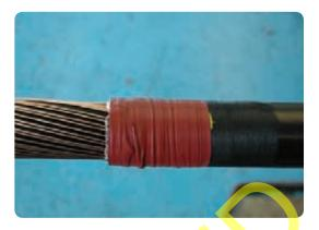
Bend back the copper screen wires carefully and lay them onto the mastic tape taking care not to cross over any of the wires. Secure the wires with a wire binder at the 60mm mark.
