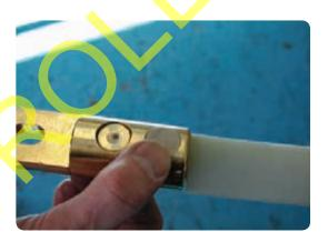
• Wrap the red sealant tape around the lug barrel, overlapping onto the insulation. Build up the diameter difference with the red tape so that a smooth and even profile is achieved.
