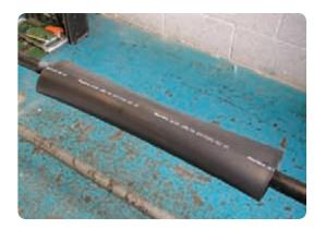
• Start shrinking the tube at the centre before working towards each end in turn. Allow to cool before moving or backfilling the joint.
