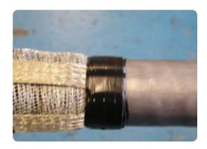
Apply one half lap layer of white fabric tape over the single-core polymeric end of the joint for a distance of 150mm from the cable oversheath to protect the tinned copper mesh tape from the heat generated by shrinking the Three-Core breakout.
