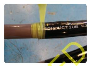
• Ensure that the bolt holes are filled with the supplied grey clay to leave a smooth profile. Use a long piece of the yellow stress control mastic to fill the ends of the connector and the insulation cut back continuing 10mm on to the insulation, and 20mm on to the connector. If there is a step between the body of the connector and the cable insulation apply yellow stress control mastic to form a smooth the profile.
