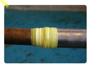
• Use a chinagraph pencil to mark the lead sheath 20mm beyond the yellow stress control tape. Position the clear barrier tubing over the core end and over the yellow stress control tape, overlapping onto the lead sheath by 20mm.
