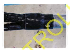
Position the short length of wrap-around heatshrink tube over the paper cable so that it
