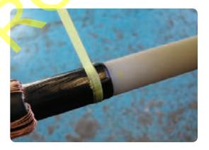
• Repeat the exercise on the paper cable core, wrapping the yellow mastic around the edge of the conductive tubing. Cover 20mm of the conductive tubing and continue on to the clear tubing for 10mm.
