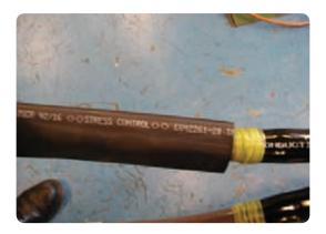
Shrink the stress control tubing down, starting from the yellow mastic tape and working towards the open core end.
