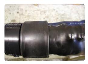
• Position the wraparound heatshrink joint sleeve around the joint and connect the two ends together using the maetal channel and the metal joining clip.
