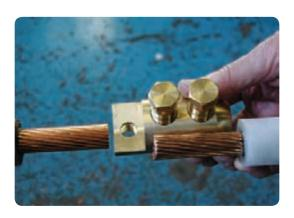
• Insert each end of the core into its respective 'connector half' and finger-tighten the bolts.
