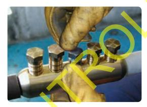
Hold the connector with the approved holding tool and tighten the two bolts on one side until they sheer off.
