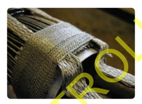
• Finally, secure the mesh and braids to the support ring and armours using the worm drive clips provided, with one clip either side of the support ring's central ridge.
