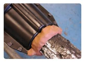
• For extra security, run a length of PVC tape down the seams of the joint shell and fit the plastic lid.
