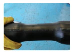
• Continue the shrinking process, working towards one end and stopping 50mm from the end. Then shrink towards the opposite end stopping 50mm from the end. Finally shrink down the first remaining 50mm of tubing followed by the second 50mm of tubing. This process ensures that no air is trapped inside the tube.
