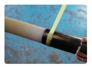
• Use the long strips of yellow stress control mastic to wrap the mastic around the connector with a 50% overlap, stretching it to about half its original width. Cover the connector area and overlap on to the insulation each side of the connector by 5mm. Make sure a minimum coverage of 2mm is achieved over the connector area.
