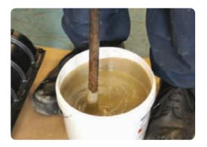
Pour the mixed resin into the joint shell.
