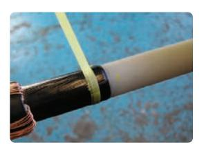
Repeat the exercise on the paper cable core, wrapping the yellow stress control mastic around the edge of the conductive tubing. Cover 20mm of the conductive tubing and continue on to the clear tubing for 10mm.
