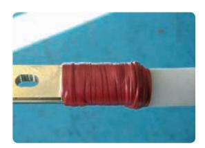
• Remove the release paper from the red tubing. Place the tubing over the cable end (with the sealant coated end downwards), level with the wire binder.
