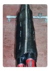
• Extra heat should be applied to the metal channel until the white marker line can be clearly seen under it.
