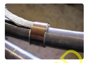
• Cover each of the roll springs with two layers of PVC tape.
