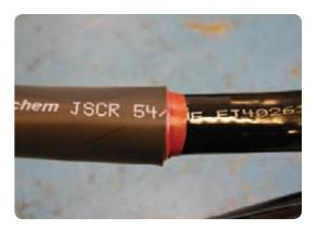
Apply one of the red mastic strips provided around the end of the stress control tube
