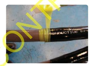
• Position a short length of the stress control tubing (54/24) over the core end, overlapping the conductive tubes and the yellow stress control mastic by 40mm.
