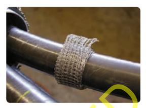
Position one of the lengths of braid over the mesh so that the loose end points away from the crutch of the cable.
