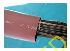
Shrink the tubing down starting at the outer sheath end, before working towards the cable lug.
