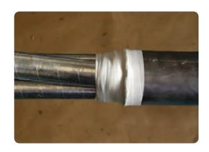
At the screen termination position wrap one layer of void filling yellow stress control mastic around each core overlapping the screen papers by 20mm and the insulation by 10mm.
