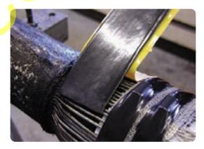
Pass the breakout over the lead sealing sleeves and pull down into the crutch. Shrink the
