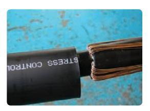
• Shrink the stress control tubing down starting in the centre, before working towards each end in turn. When finished the tubing should be fully shrunk and wrinkle free.
