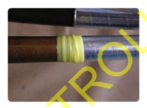
• Slide the clear barrier tubing over each core and position 30mm from the end of the metal sheath. Shrink down the tubing starting at the crutch position before working towards the open core ends. Check the tubing is shrunk down evenly and is free from creases or wrinkles.
