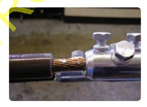
Check that the connector butts up against the insulation and finger-tighten the bolts.
