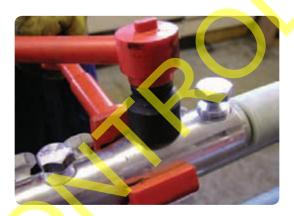
• Smooth off any sharp edges from the bolts and then clean and degrease the connector. Fill the bolt holes with the supplied grey clay to obtain a smooth finish.
