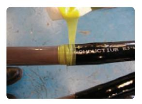
• Check that the bolt holes are filled with the supplied clay to leave a smooth profile. Using a long piece of the yellow stress control mastic, fill the ends of the connectors and the insulation cut backs, continuing 10mm on to the insulation and 20mm on to the connector. If there is a step between the body of the connector and the cable insulation apply yellow stress control mastic to form a profile.
