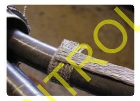
• Secure a length of earth braid to each lead of the lead sheaths using one turn of the roll springs directly on to the copper mesh wrap.
