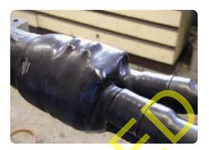
Position the crutch sealing sleeve with one end level with the end of the fingers on the breakout and shrink into place.
