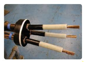
Position a combined tube set (stress control, insulating tube and screened insulating) over each of the single-core polymeric cables.
