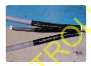
• Slide the small yellow mastic wedge into the crutch using the installation tool provided. Take the larger wedge and insert it into the crutch behind the smaller wedge using the same tool. Remove the nylon tape after insertion of both wedges.
