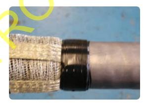
Wrap the remaining exposed lead sheath with the strips of red sealant tape. This is an important moisture seal. Do not leave out.
