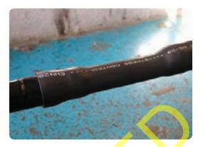
• Wrap a piece of red sealant mastic around each end of the stress control tubing. Start from 10mm on the stress control tubing and extend for 10mm onto the core screen at both ends.
