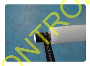
• Increase the conductor diameter sufficiently so that the insulating rod is a snug fit over the conductor. Push the insulating rod onto the conductor ensuring that it butts against the cable insulation.
