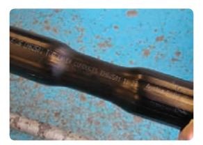
Continue to shrink the tube from the centre to within 50mm of one end.
