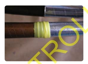
• Slide the clear barrier tubing over each core and position 30mm from the end of the metal sheath. Shrink down the tubing starting at the crutch position working towards the open core ends. Check the tubing is shrunk down evenly and free from creases or wrinkles.
