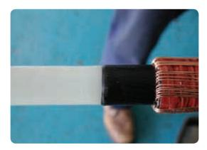
Make a mark with a chinagraph pencil 20mm on to the core screen and 10mm on to the insulation.
