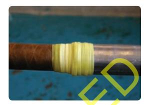
Make a mark on the lead sheath using a chinagraph pencil 20mm beyond the yellow stress control tape. Position the clear barrier tubing over the core end and the yellow stress control tape overlapping onto the lead sheath by 20mm.
