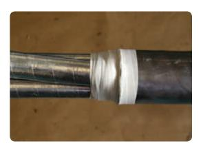
• At the screen termination position wrap one layer of void filling yellow stress control mastic around each core, overlapping the screen papers by 20mm and the insulation by 10mm. Remove the metal binder from the screen edge during the taping process.
