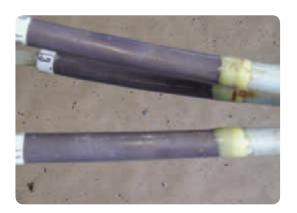
Slide the black conducting tubing over the core ends and position them 50mm from the end of the metal sheath. Shrink the tubes down at this position starting at the crutch working towards the core ends.
