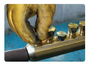
• Using the approved insulated tool to hold the connector, take up the tension on all the bolts equally without shearing them off.
