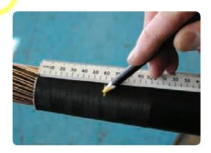
• Wrap one layer of red sealant tape over the cable sheath down to the chinagraph pencil mark.
