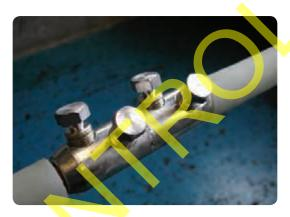
• Using the approved insulated tool to hold the connector, take up the tension on all the bolts equally without shearing them off.
