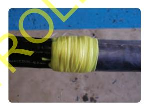
Pass the conductive breakout over the cores and push it well down into the crutch, using
