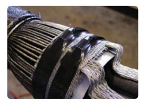
• Slide a sealing sleeve over each lead sheath and roll spring connection up to where the earth braid meets the support ring. Shrink them down starting on the lead sheaths and continuing towards the armour wires area.
