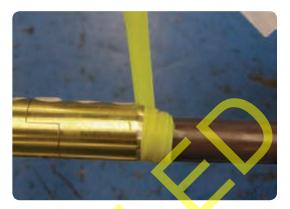
• Remove the release paper from one of the yellow stress control mastic patch and wrap it centrally around the connector, taking care to exclude the air as it is wrapped. When finished the patch should be smooth and wrinkle free. Repeat the process with all three connectors.
