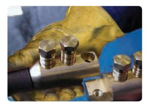
Align and position the two connector halves so that the central fixing bolt can be inserted
