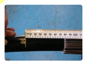
• Remove the insulation for 30mm from the end of the cable.
