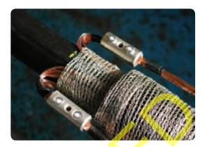
Wrap a second layer of the copper mesh around the joint, as before, so that the whole
