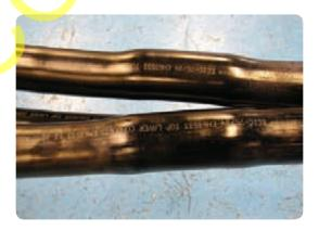
Position the three compression sleeves over the paper end of the joint, so that they equally overlap the red and black insulation tubes and the core tubes. The uncoated end of the compression sleeve should be positioned towards the centre of the joint. Shrink in place starting from the centre of the tubes towards the centre of the joint before finally shrinking from the centre towards the crutch.
