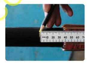
• Remove the core screen down to the 40mm mark using the approved screen stripping tool.
