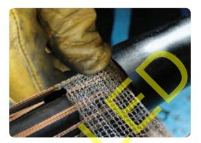
• Continue across the whole joint with the tinned copper mesh at a 50% overlap and secure on to the opposite joint side.
