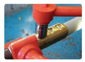
• Clean and degrease the connector. Fill the bolt holes with the supplied grey clay to obtain a smooth finish.
