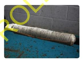
• Clean and degrease the outer sheaths of both cables for 150mm from the sheath cut. Slide the large outer sealing sleeve centrally over the joint area.
