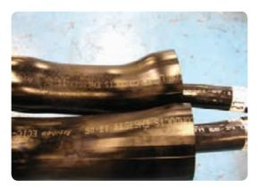
• Remove the heat from that end and start shrinking from the middle again towards the other end of the tubes. Stop again 50mm from the end. This ensures air inside the tube is expelled as the tube shrinks.
