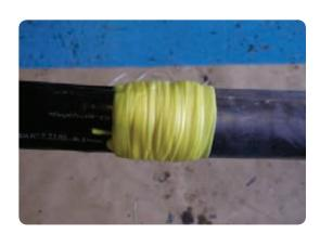
Pass the conductive breakout over the cores and push it well down into the crutch, using the yellow wedge installation tool. Hold the breakout in place and shrink it down starting at the centre, before firstly working towards the lead sheath and then towards the breakout fingers.
