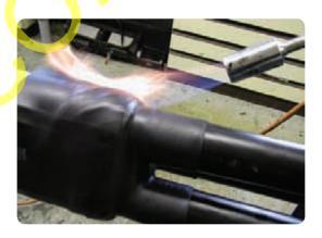
• Wrap the remaining exposed lead sheath with the strip of black mastic sealant tape. This is an important moisture seal. Do not leave out.
