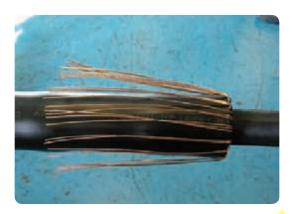
• Wrap the tinned tinned copper mesh with a 50% overlap around the pot end, starting at the outer sheath and continuing up onto the copper screen wires, before covering the insulating rod.
