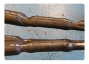
• Remove the release paper from one length of the red sealant mastic tape and wrap it around the end of the stress control tube. Overlap the tape on to the tube by 20mm and by 10mm on to the core.
