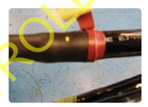
Position a short length of the larger diameter stress control tubing (54/24) directly over the
