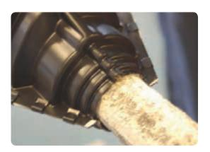
Tape the joint box to the incoming cable with PVC or another suitable tape. If large gaps
