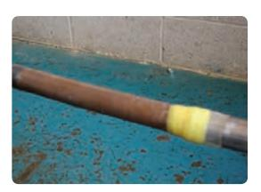
• Position the short black conductive sleeve 220mm from the core end and shrink the tubing down, starting at the open cable end before working towards the lead sheath.
