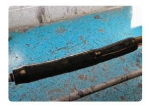
• Pull the black compression sealing sleeve across the joint to the paper cable side and place it so that at least 50mm of lead sheath is still visible.
