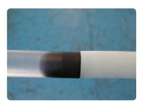
• Use a short strip of yellow stress control mastic and remove the release papers from a short strip of yellow stress control mastic tape. Wrap it around the edge of the insulation screen starting 20mm from the screen edge, before continuing for 10mm on to the core insulation. Stretch the tape to approximately half its original width to obtain a fine edge onto the insulation.
