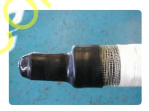
• Check that the over-sheath is clean and degreased. Position the outer sealing sleeve over the pot end assembly so that it lines up with the end of the end cap.
