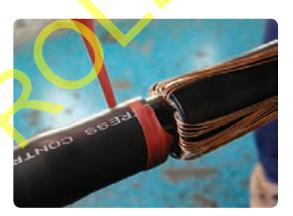
Pull the red insulating tubing from inside the nested tube set and position it centrally over the stress control tube. Start shrinking in the centre before working towards each end in turn.
