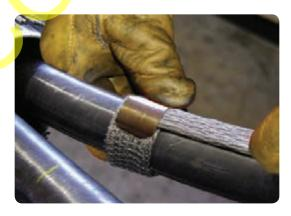
• Bend the braids back over the roll spring and then secure in place with the remaining turns.
