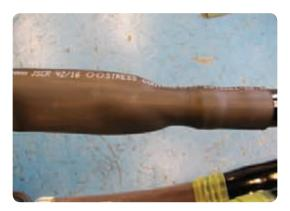
• Wrap one of the red mastic strips provided around the end of the stress control tube 30mm on to the tubing and 10mm on to the core.
