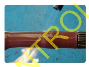
• Place the black and red screened insulating tubing over the assembly and position it to coincide with the previously installed tubes.
