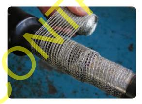
Lay the copper screen wires back across the joint and form them into three separate earth conductors. Connect the copper screen wires to each of three earth braids using mechanical connectors provided in the kit.
