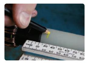
• Stretch one of the short yellow stress control mastic supplied in the kit to half its original width. Wrap it around the core screen and insulation between the two chinagraph pencil marks. Repeat for the other cable side.
