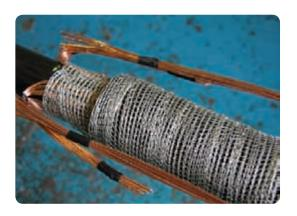
Gather the wires together and cut them centrally above the tinned copper mesh overlapping the cable sheath. Install the copper screen wire conductors into their respective connector and tighten the bolts until the heads shear off.
