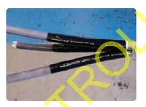
Slide the smaller supplied yellow mastic wedge into the crutch using the installation tool
