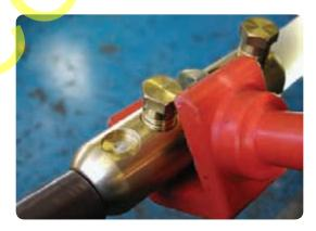
• Repeat the operation on the other side of the connector. Check that the combined tube set is located over the single-core cables and sheer off the central fixing bolt.
