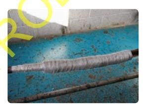
• Fold back the copper screen wires over the joint and form them into an earth lead except for the area over the lead sheath. At this point open up the wires and place them directly on to the tinned copper mesh. Wrap the roll spring over the screen wires and twist up tight.
