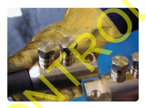
• Fit the conductors into the connector. The insulation should butt against each end of the connector.
