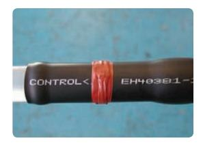
• Slide the red insulating tubing over the stress control tube butting it against the cable oversheath and coinciding with the stress control tubing edge.
