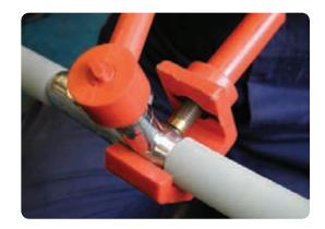
Continue to tighten and sheer off all the bolts starting with the bolts at each end followed by the central bolts.
