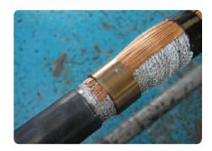
Completely cover the roll spring with two layers of PVC tape.
