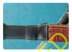
Remove the insulation from the core end according to the inner dimension of the cable lug barrel.
