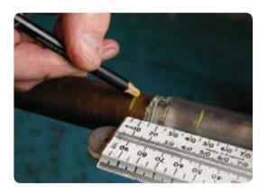
• Remove the release paper from one of the medium lengths yellow stress control tape. Stretch the tape to about half its original width and wrap it around the lead sheath for 20mm. Remove the twine binder from the screen edge and continue with the tape over the screen papers and on to the insulation for 10mm.
