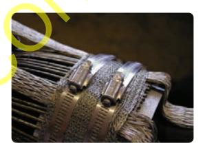
• Cover the worm drive clips with PVC tape to tidy up their loose ends.
