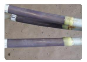
• Slide the black conducting tubing over the core ends and position them 50mm from the end of the metal sheath. Shrink the tubes down at this position starting at the crutch before working towards the core ends.
