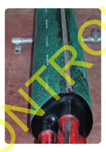
• Shrink the wraparound sleeve in place, starting at the middle before moving towards each end in turn. The green paint on the surface of the sleeve should disappear when the tube is correctly shrunk.
