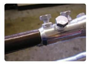
• Insert the single-core polymeric cables into the connector ensuring that the connector butts up against the insulation and finger-tighten the bolts.
