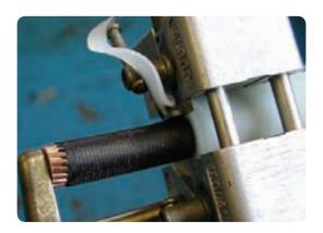
• Remove the tool and the insulation spiral. Carefully remove the remaining conductor screen using an approved knife.
