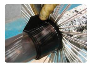
• Make a mark with a Chinagraph pencil 130mm from the end of the outer sheath. Wrap a length of copper mesh around the lead sheath up to the 130mm mark.
