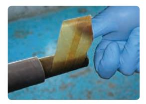
Clean any surplus compound from the cable conductor with an approved wipe.
