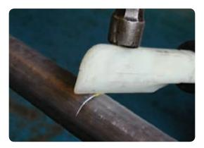
• Cut the lead sheath across from the open cable end to the circular cut. Use an appropriate approved hack knife. Take care not to damage the Copper Woven tape below.
