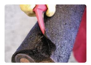
Remove the binder and lift the armours with an approved hack knife so they are 90° to the
