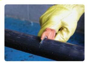
• Now make a lengthwise cut along the sheath towards the sheath cut position taking care not to damage the underlying lead sheath.
