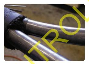
• Build up the remaining inner bedding using the black mastic from the Three-Core transition joint and the HSL module to suit the support ring's inner diameter. Fit the support ring over the build up tape, positioning it 60mm from the uplifted armours.
