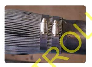
• Apply a layer of PVC tape to the worm drive clips to cover any sharp edges. Position the armour sealing sleeve 30mm beyond the armour edge and shrink down starting at the lead sheath end before proceeding towards the cable over-sheath.
