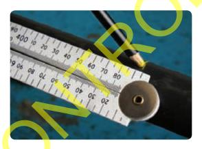
Make a circular cut at this mark using an appropriate approved tool. Check that the cut is only three quarters through the sheath thickness.
