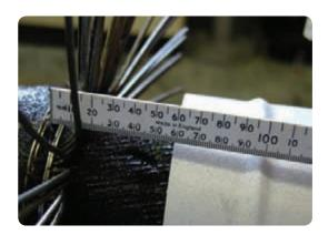
• Wrap the length of supplied black mastic behind the support ring, butting it against the armours wires. Lay the armours down onto the ring and secure them with a wire binder.
