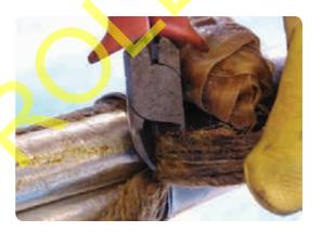
• Rewind the CWT tightly around the cable cores at the crutch position for a distance of 20mm from the lead sheath, then cut and tie off. Remove any surplus tape with insulated side cutters.
