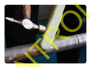
• Open the lead sheath up along the length of the cut and carefully unwrap the lead sheath against the ring cut.
