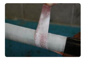
• Clean and degrease the insulation with an approved solvent wipe to remove all traces of any remaining loose material. Always wipe from the open core end towards the screen wires to avoid contaminating the insulation with carbon from the remaining screen.
