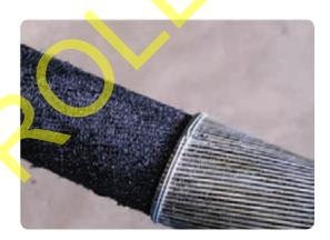
• Remove the binder and lift the armours with a hack knife so they are 90° to the cable. Clean off all traces of bitumen from the wires using a gas torch and approved solvent wipes.
