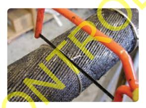
Wear suitable gloves while removing the armour. Lift and unwrap the armour wires a few at a time and break them off against the binder by bending them backwards and forwards.
