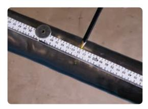
Wear suitable gloves for this operation. Use an approved hackknife to make a circular indented ring cut around the lead sheath at the pencil mark, taking care to only cut part way through the sheath.
