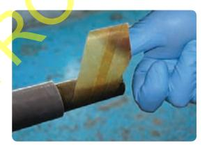
Clean any surplus compound from the cable conductor with an approved solvent wipe.
