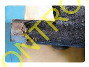
Apply more heat to the final layer of bitumen on the lead sheath and armours and wipe
