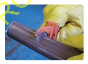
Remove the clear barrier tube by pulling towards the end with a gentle twisting movement.
