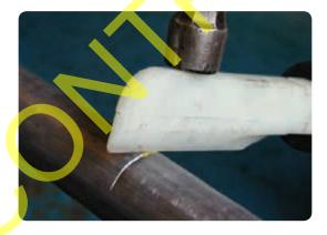
• Cut the lead sheath across from the open cable end to the circular cut. Use an appropriate approved hack knife. Take care not to damage the Copper Woven tape below.
