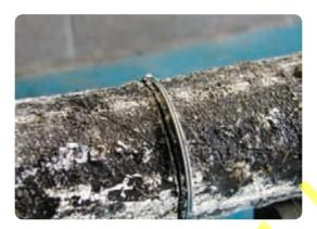
Remove the serving with the approved knife and heat from a gas torch if required or in the case of a polyethylene sheath use the approved tool for this operation.
