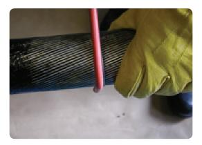
• Wear suitable gloves while removing the armour. Lift and unwrap the armour wires a few at a time and break them off against the binder by bending them backwards and forwards.
