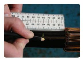
Smear a thin coating of Silicone grease over the conducting screen layer. Starting at the
