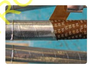
• Remove the numeral paper and one layer of paper below to the same point as the screen papers, using the same method and marking the cores with the matching numbered phase tape.
