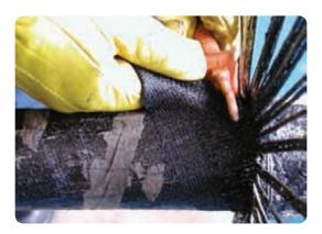
At the open cable end lift the bitumen impregnated textile layer with a knife and unwrap it back to the vertical armour position, tearing it against the score previously made. The use of a gas torch may assist this process.
