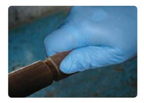
Unwrap the papers up to the cut position and tear off neatly against the barrier tube edge.
