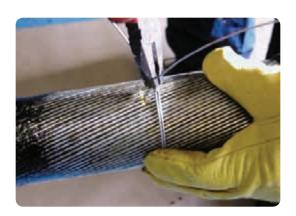
• Using an approved saw, make a circular cut around the armours at the binder position. Cut through only half the width of the armour to avoid damaging the lead sheath below.
