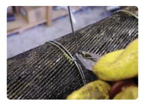
• Using an approved depth guarded or junior saw make a circular cut around the armours at the binder position. Cut through only half the width of the armour to avoid damaging the lead sheaths below.
