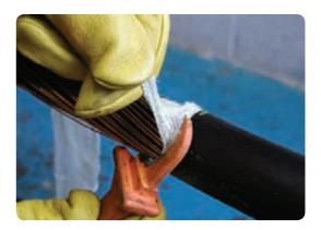
• Unwind the copper wires and lay them back along the over sheath in the position required by the joint being made and secure with PVC tape. If preparing for a termination a length of red mastic sealing tape should be applied to the outer sheath following the appropriate instruction.
