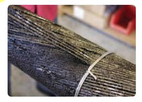
At the open cable end lift the bitumen impregnated layer with a knife and unwrap it back to the armour cut position. Remove it at this point, taking care not to damage the underlying lead sheaths.
