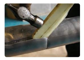
• Open the lead sheath up along the length of the cut and carefully unwrap the lead sheath against the ring cut.
