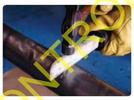
• From the open cable end, cut the lead sheath longitudinally to the circular cut using the appropriate approved hack knife. Take care not to damage the Copper Woven Tape (CWT) below.
