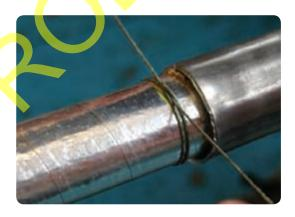
Unwrap the screen carefully to the termination point and remove it by neatly tearing against
