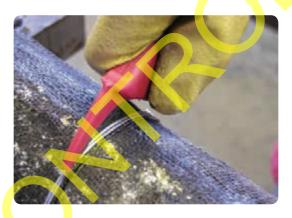
• Remove the serving with the approved knife and heat from a gas torch if required.
