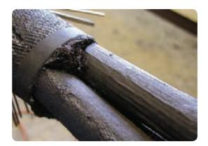
• Apply more heat to the final layer of bitumen on the lead sheaths and wipe off all traces of bitumen with the approved solvent wipes.
