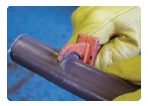
• Lift the edge of the sheath and unwrap along its length, tearing off at the circular cut point. The use of a gas torch may assist this operation if necessary.
