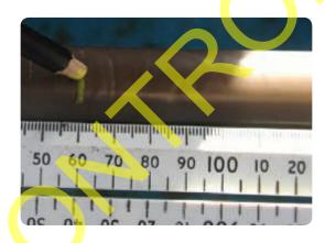
• Using a sharp knife cut around the core and through the papers taking care not to damage the conductor below.
