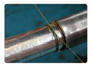
• Unwrap the screen carefully to the termination point and remove it by neatly tearing against the twine binder. Remove any carbon paper below the screen to the same termination position, followed by two of the insulation papers.
