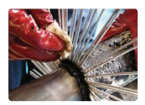
Apply two wraps of black mastic sealant around the lead sheath butting up against the raised armours.
