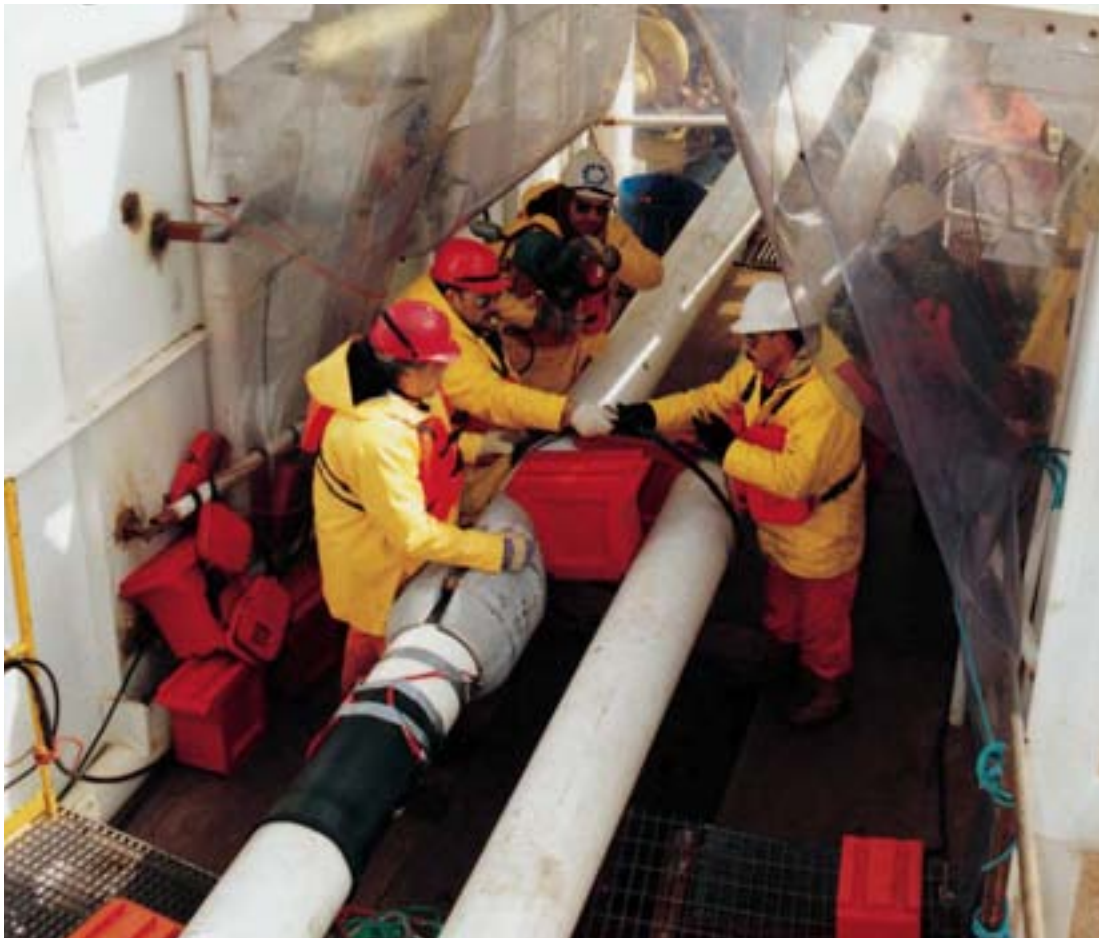
Dual Lay Pipeline Spacers with Metallic Banding installed on Lay Barge
