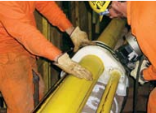
Banding being installed onto the blocks on the Lay Barge
