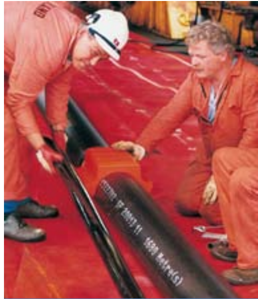
Installation of Bundle Clamp
