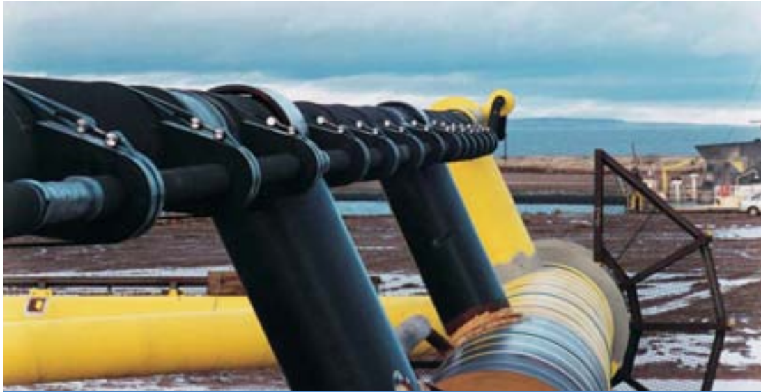
Riser Clamps complete with Kelvar Straps installed on platform
