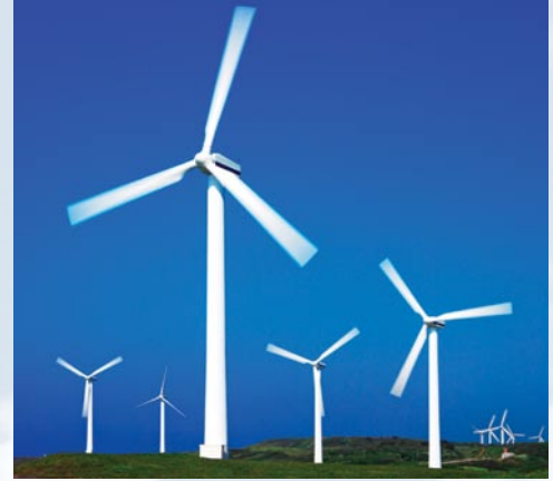
A modern wind turbine is designed to operate for more than 20 years, with an average 45–50 RPM. T&B designs its products to exceed this life expectancy.
