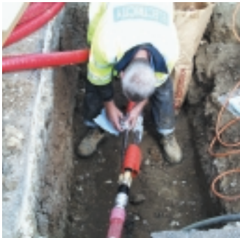
Connector installation
