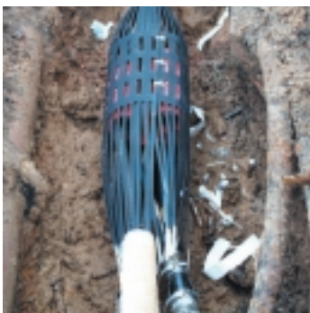
Earth cage installation
