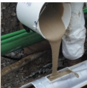
Filling the completed joint with Polyurethane resin
