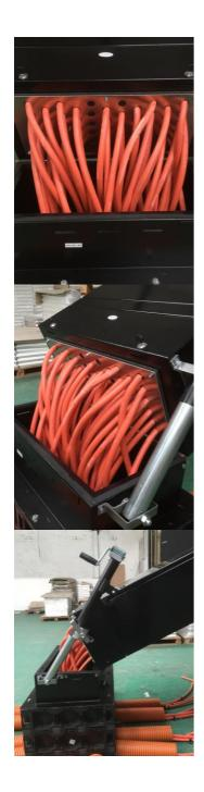
The Ritherdon Hinged Controller Base (HCB) provides easy access for cable installation, removal or replacement from signal cable ducting into a controller cabinet.
