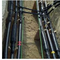
Heat-shrinkable joints for polymeric cables up to 72 kV
