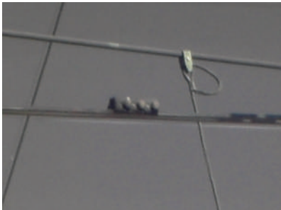
Contact wire splice
