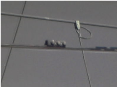
Contact wire splice
