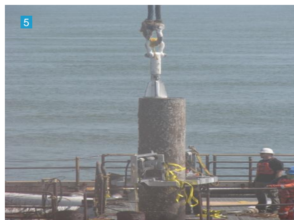
Conductor lifted to the surface
