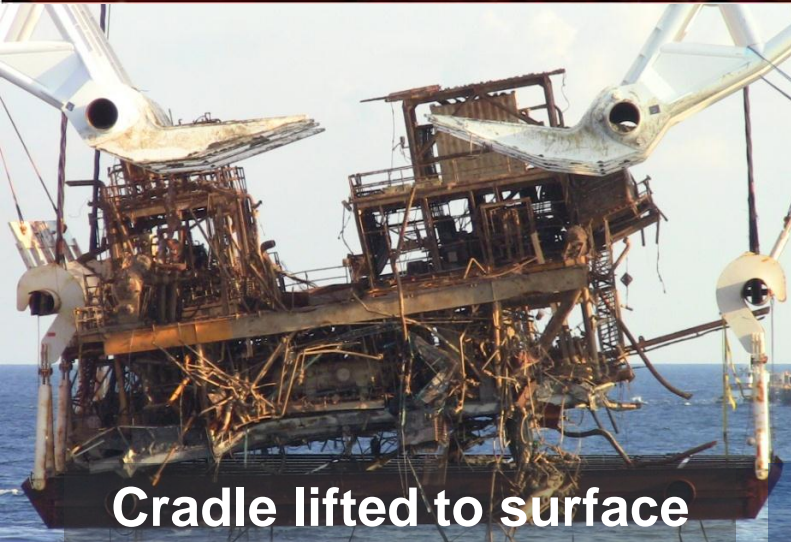
Claw lifting deck to cradle
