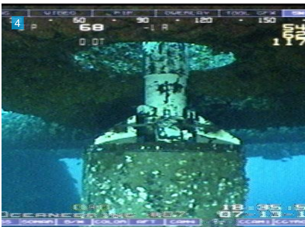
Conductor lifted through conductor guide
