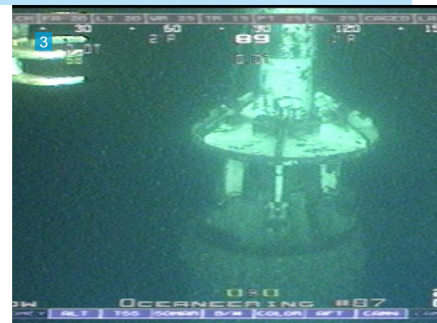
Spear entering well conductor
