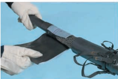
Applying sealing mastic
