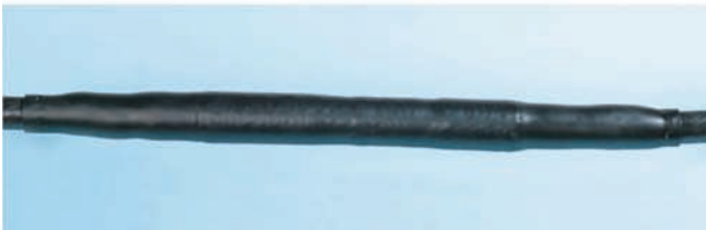
The completed installation
