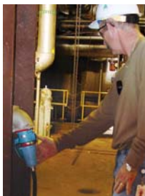
Portable equipment connection
