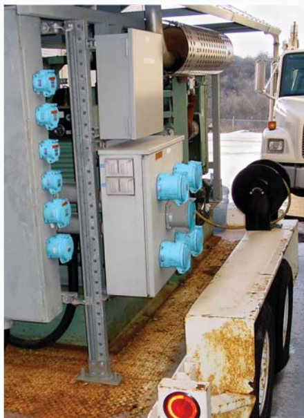
A mobile diesel generator supplies power via Marechal plugs & socket-outlets during outage conditions.
