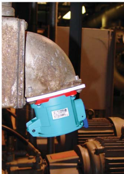
Modular construction made it simple for this power plant to convert their existing pin and sleeve socket-outlets to Decontactors.
