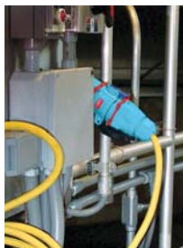
Wastewater mixer connection
