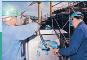
Supply to building sites (shipyards)
