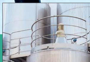
Power supply to motors and pumps
