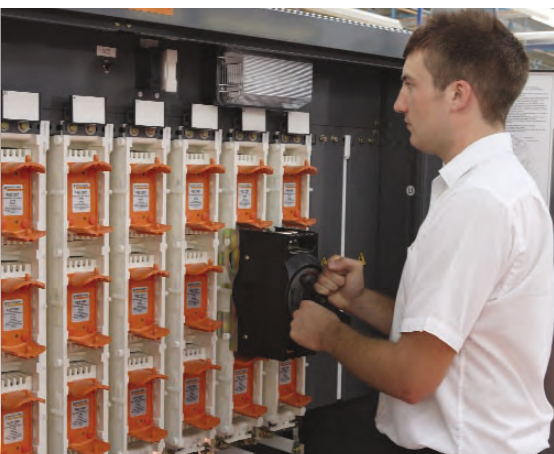
▲ Safe switching at a SAIF feeder pillar
