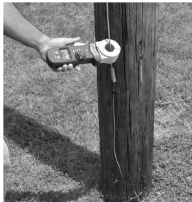
The Megger DET20C clamp-on ground tester is shown being used to test a utility pole
