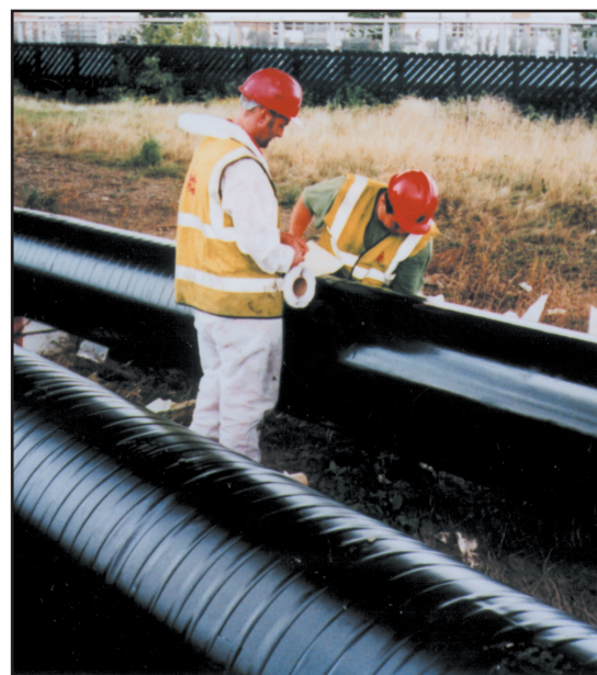
Hand wrapping pipe lengths with Densoclad Tape.
