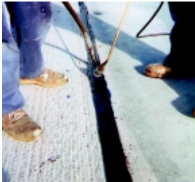
Application to asphalt/concrete airport runway.
