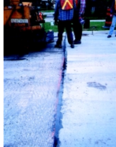
Application to asphalt/asphalt road repair.
