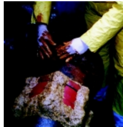
Application of Petrolatum Tape system.
