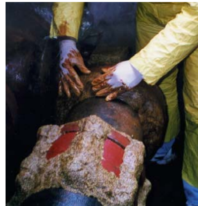
Application of Petrolatum Tape system.
