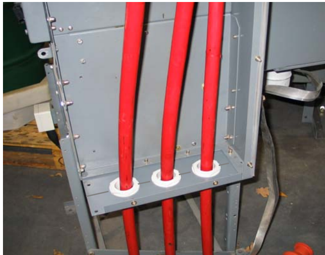
Completed installation (termination or earthing not shown)
