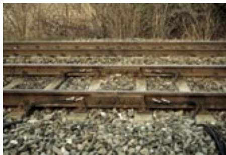
Connection of metal structures to rails for earthing purpose
