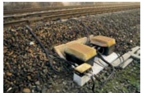
Connection of metal structures to rails for earthing purpose
