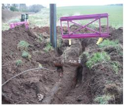
Even if you scan an area thoroughly using a cable locator in both power and radio modes you will more than likely not pick up a signal from a street lamp cable when the street lamp is not switched on. It is therefore important that you are aware of your surroundings and make note of any obvious areas where a cable will be buried e.g. the area surrounding a street lamp. If you excavate without this kind of care you are endangering your life, your colleagues' lives and your equipment.
