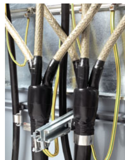
Mounting two 3-core cables with screen connection kits and three 1-core cables
